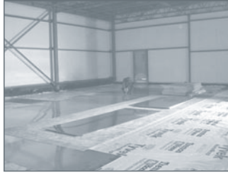
Installing the floor in the new penthouse (top) level in January, 2010
