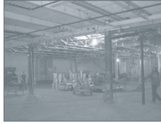
Progress of internal construction (one level of three) in May, 2010
