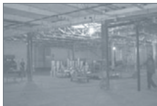
Progress of internal construction (one level of three) in May, 2010
